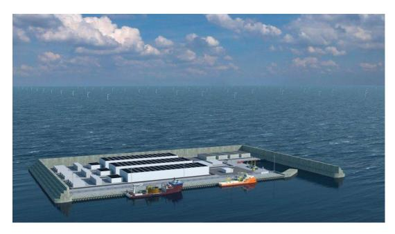
The initial giant island 120,000 m<sup>2</sup> (may grow to three times the size) some 80km from Denmark's shore will provide enough energy for three million households from 200 giant offshore wind turbines, each some 260m high.
