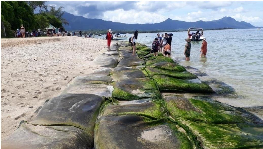
Figure 14 Sandbags placed to address coastal erosion
