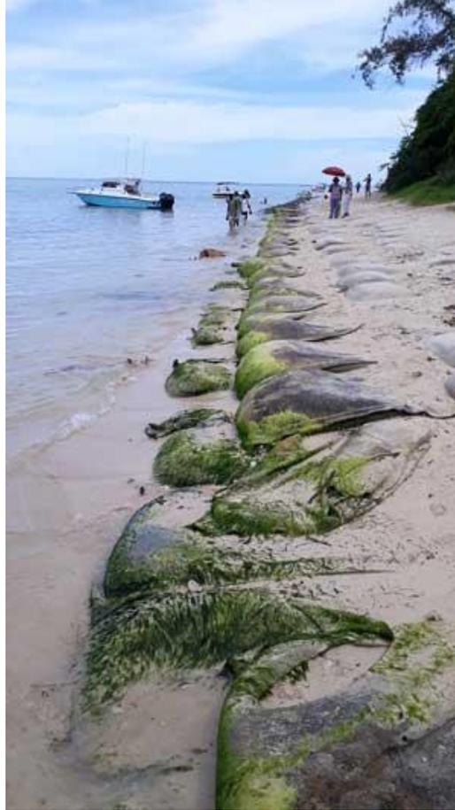
Figure 15 Gradual degradation of the sandbags-state after about 2 years
