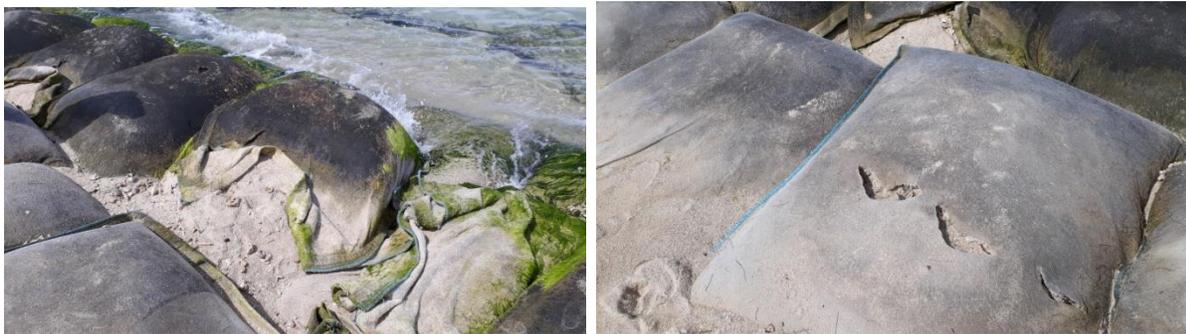
Figure 2. Damage to sandbags due to wave actions and human trampling
